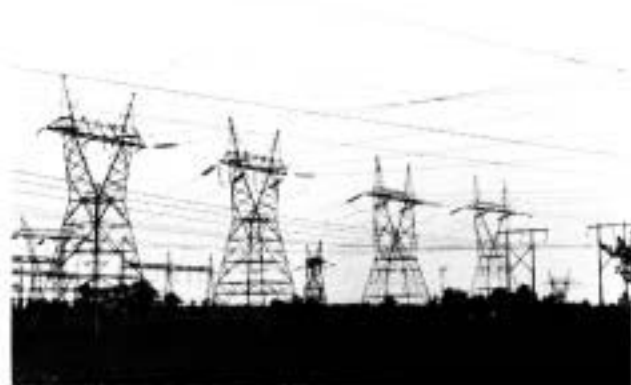
Figure 1. The confluence of four 345 kV transmission lines in Clay, New York.
